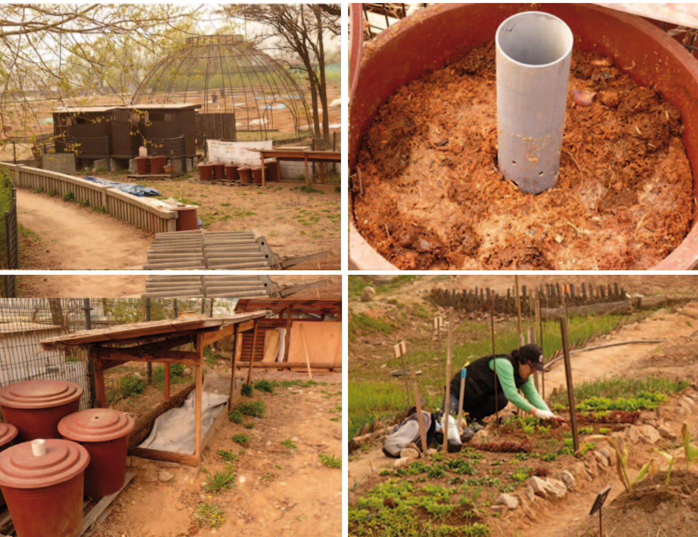
Figure 6.2: A sanitation facility in a public community garden in Seoul with fermentation pots and devices for humification by worms.
