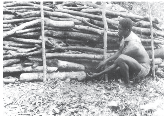
Figure 2.9: Combination of mound and pit kiln (Food and Agriculture Organization 1983).
